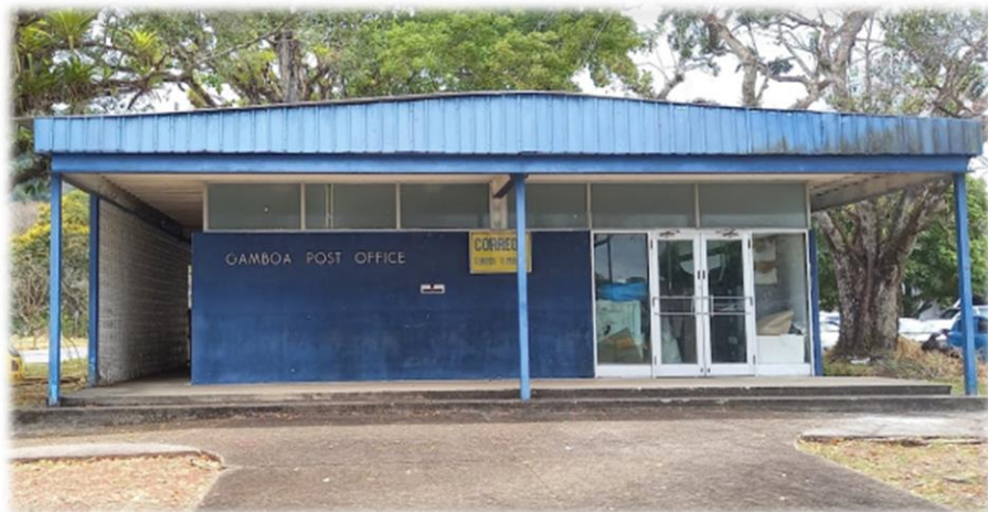
Post Office (abandoned)
