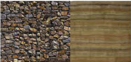
The Old Souk uses Gabion and Rammed Earth walls in both architecture and the streetscape.
